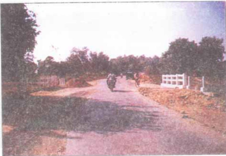
WODC Funded Project - Widening to the existing narrow culvert at 1st k.m.
