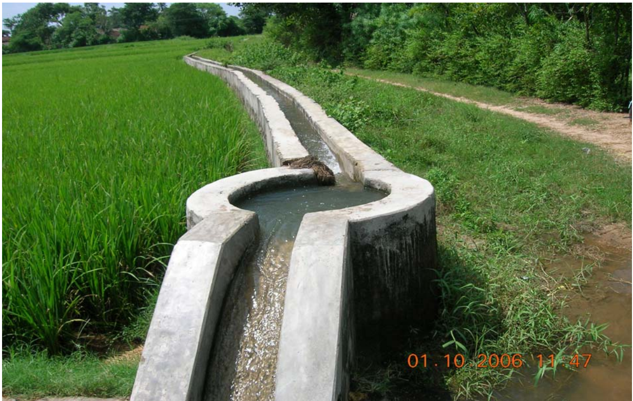
Photograph – 10: Field Channel of lift project of OAIC in Binka, Sonepur
