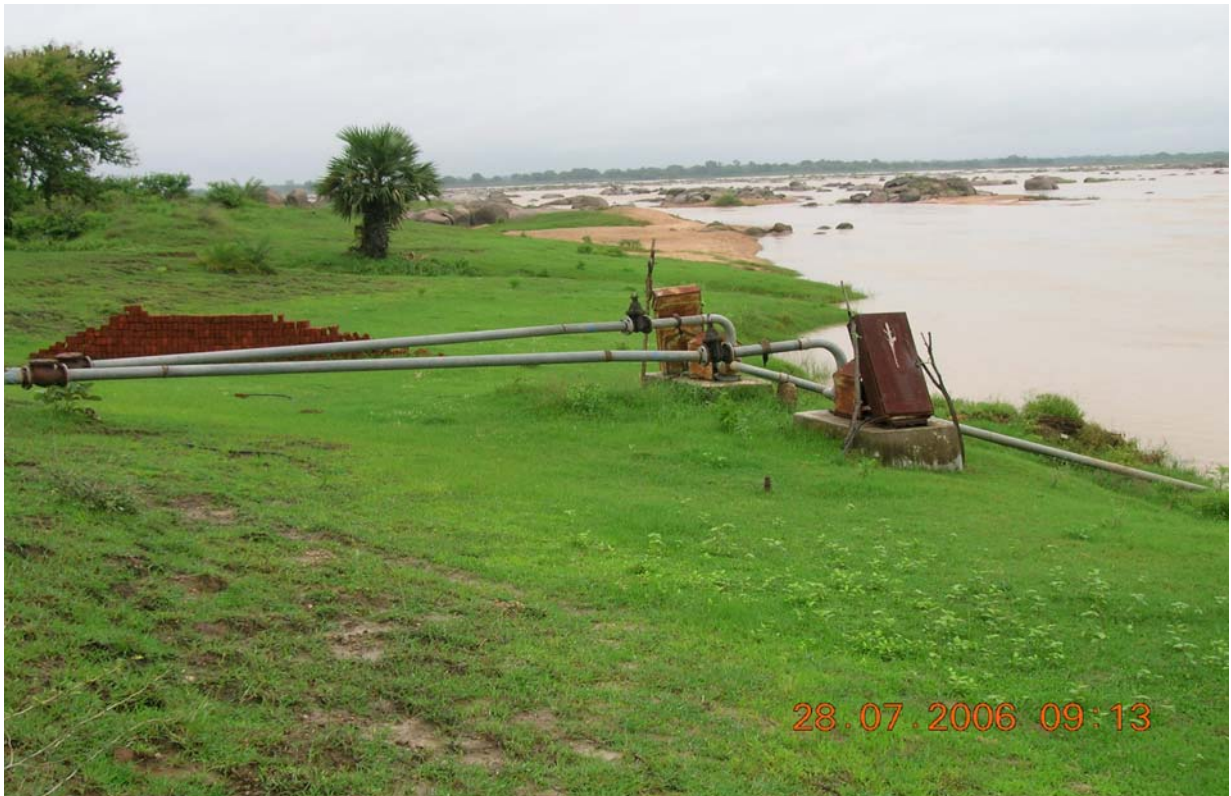
Photograph – 4: BKVY Lift Point of OLIC at Sonapur
