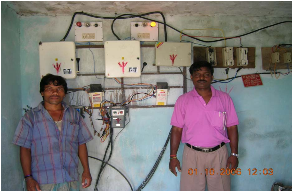
Photograph – 6: BKVY Pump house of OAIC in Binka, Sonapur
