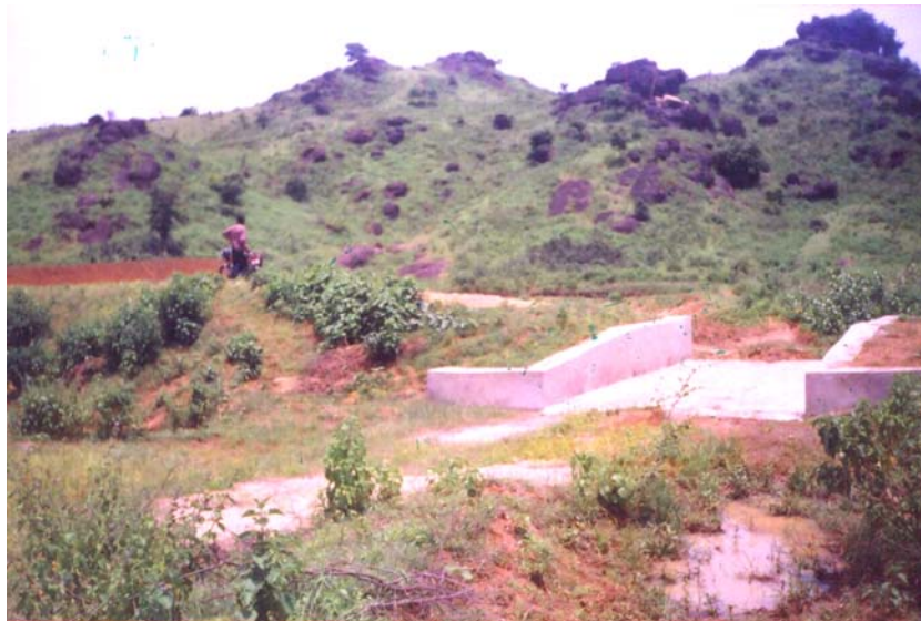
Dukurigudi Micro-Watershed Goudtala Masonary Surplus, Kalahandi; Collecting surplus rain water for agriculture and ground water recharge.
