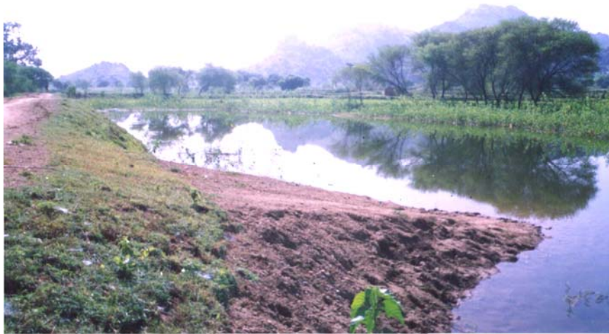
Run off Management Structure (Guide Bond -1) Goudtala
